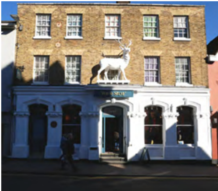
Figure 22 – this retailer now has a unique presence in Bishop's Stortford with a subtle fascia.
