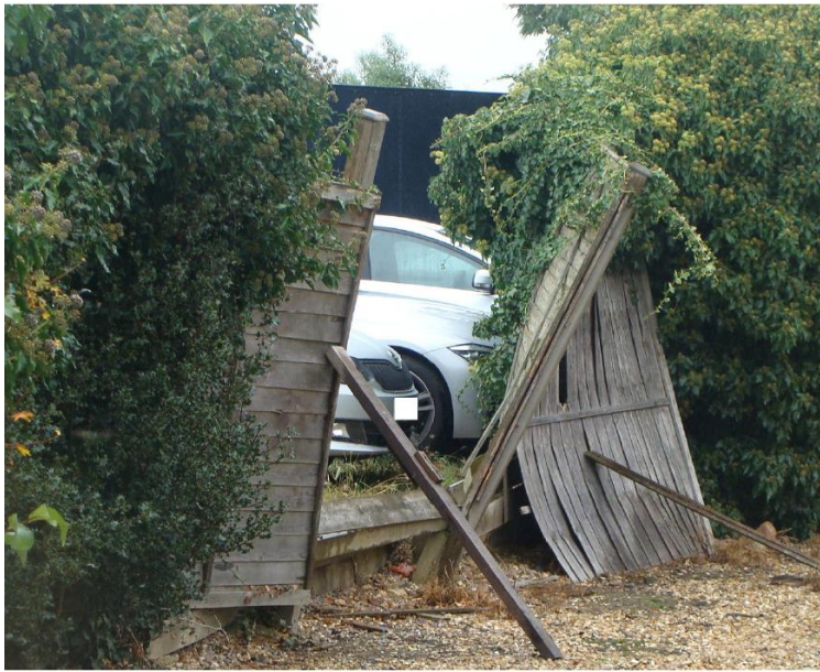
Picture. Broken boundary fence between No. 1 Buryfield and adjacent PH detracts. The owner has promised a positive outcome.
