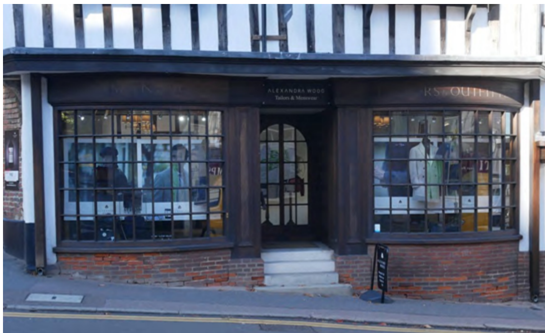
Figure 9 – a 15th century timber-framed house converted to retail use on the ground floor. The shopfront dates from the early 20th century and is of an appropriate design.
