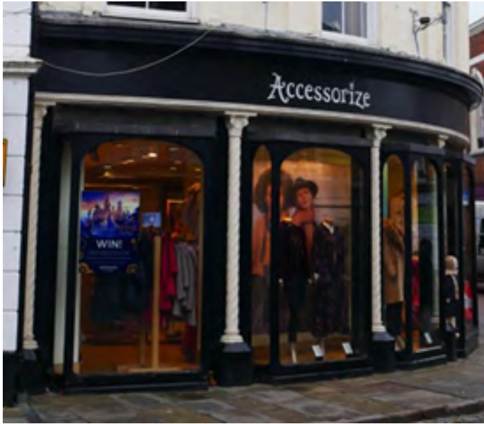
Figure 21 – The identity of a chain store respecting the style of the curved shop with its fascia supported on barley twist columns with plinth and ornate capital.
