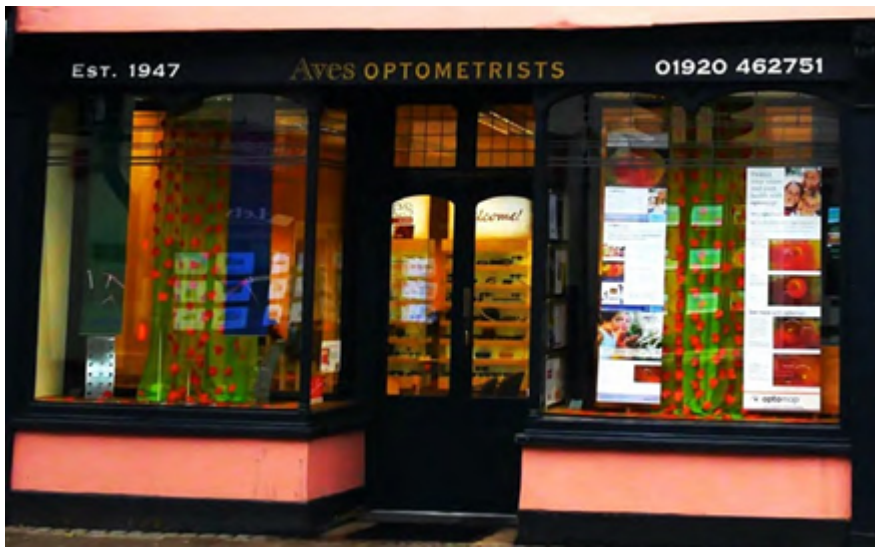
Figure 36- Appropriately scaled lettering to height of fascia.
