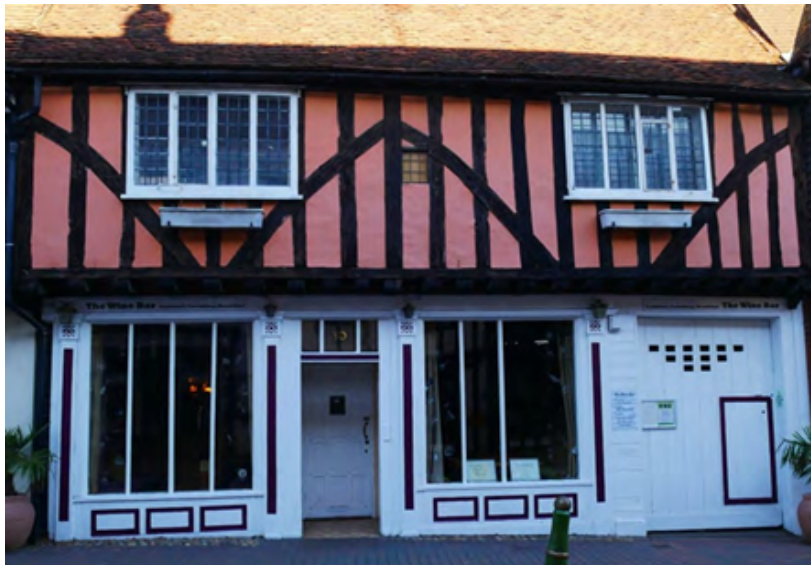
Figure 1 – Formerly a house but adapted to provide a double fronted shop to the ground floor.
