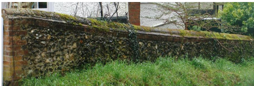
Picture 23. Wall of brick and flint construction to front of Clare Cottage Snow End House .
