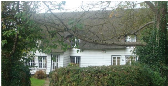
Picture 10. Well Cottage one of a number of important thatched properties in the local street scene.
