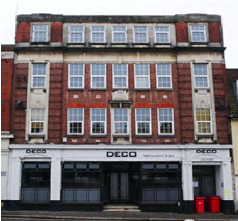
Figure 19 - Neo-classical revival building with defined fascia and architectural features.
