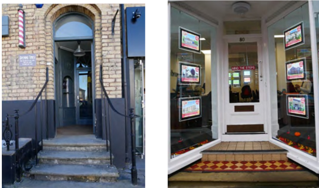
Figure 46 - A historic entrance with original handrails assisting entry (left). An additional step to ease entry (right), however a uniform surface treatment would have been more appropriate.
